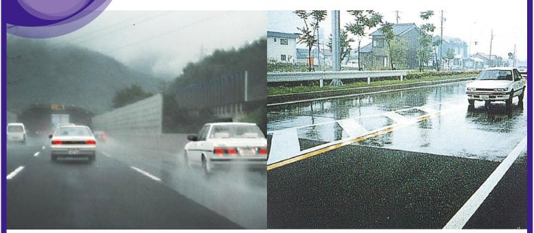
This pavement functions to drain rainwater and other water accumulations to the roadside or shoulder without stagnating on the road surface.
